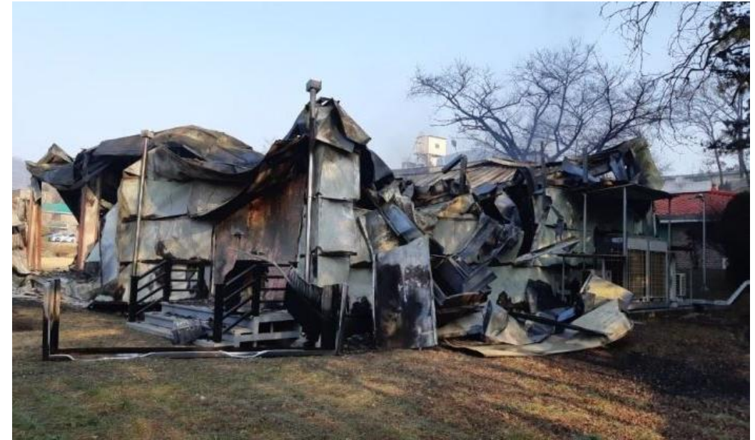
Site of Battery Fire in South Korea (Source: Korea Times)
