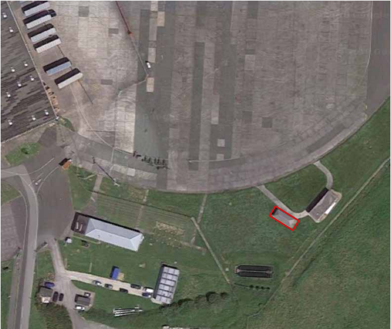
Figure 6. Aerial view of St Columb Major substation (437490) outlined in red on the Aerohub site. (Source: Google and the Google logo are registered trademarks of Google Inc., used with permission)
