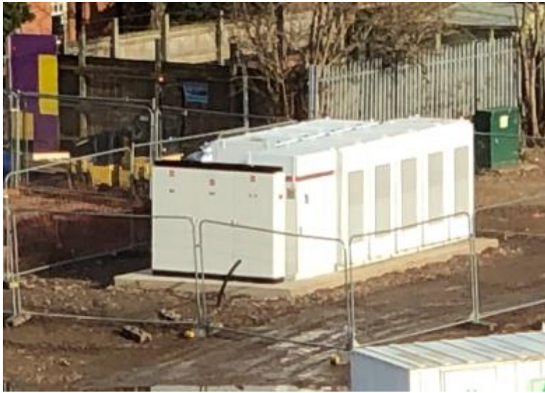
Tesla 2.1MWh Battery - 500kW inverter
