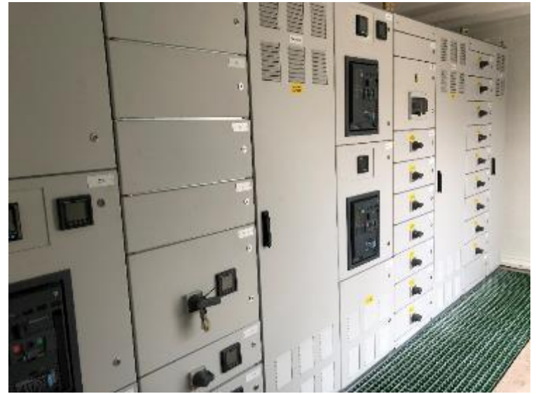
Low Voltage Distribution Panels
