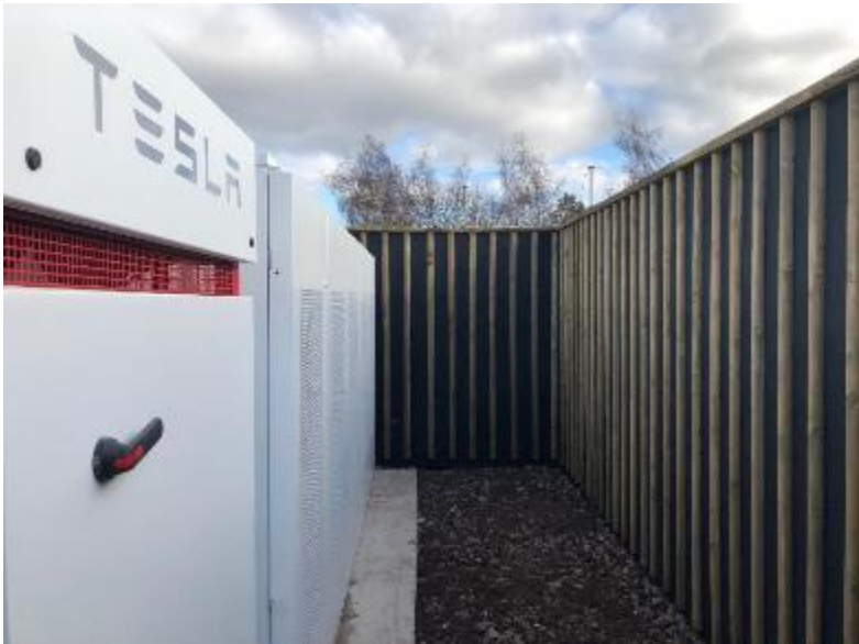
Enclosure - Security and Acoustic Fencing
