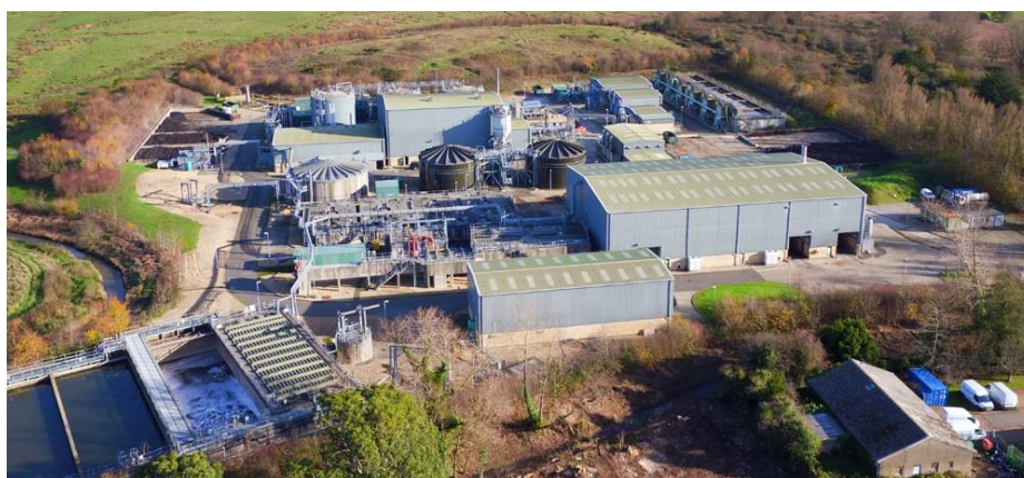
Figure 50: Aerial view of Sandown Sewage Treatment Works | Credit: Island Echo, September 2021
